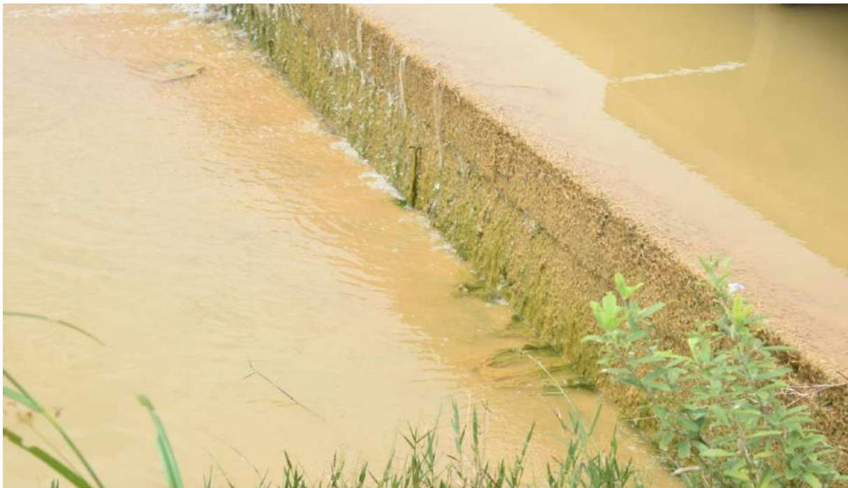
Figure 34: Algae growth noted along the stepping stones in Elmina Central Park.
