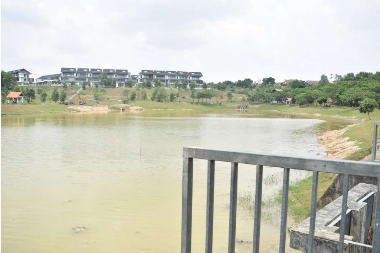
Figure 7: Current condition of Pond C.
