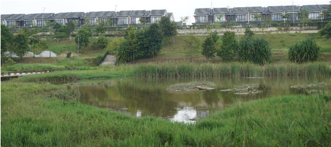
Figure 63: Accumulation of sediment formed small islands after long overdue maintenance
