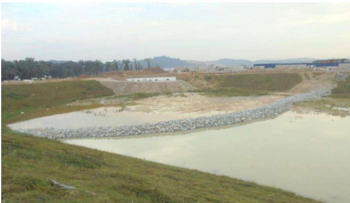
Figure 50: An example of sediment forebay at Pond 2.
