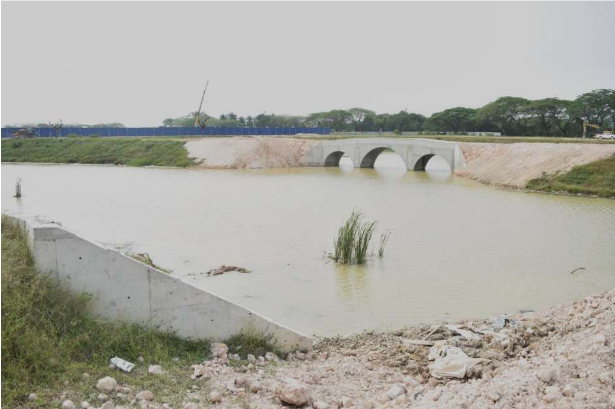
Figure 17: Pond 2 still under construction.
