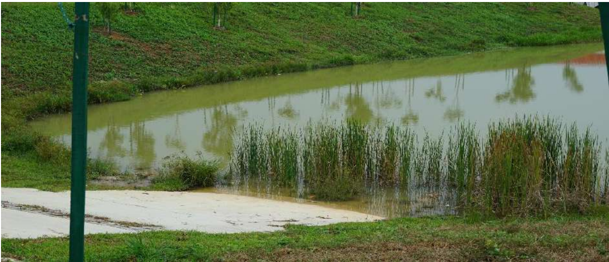
Figure 56: An example of maintenance access from Pond 2.
