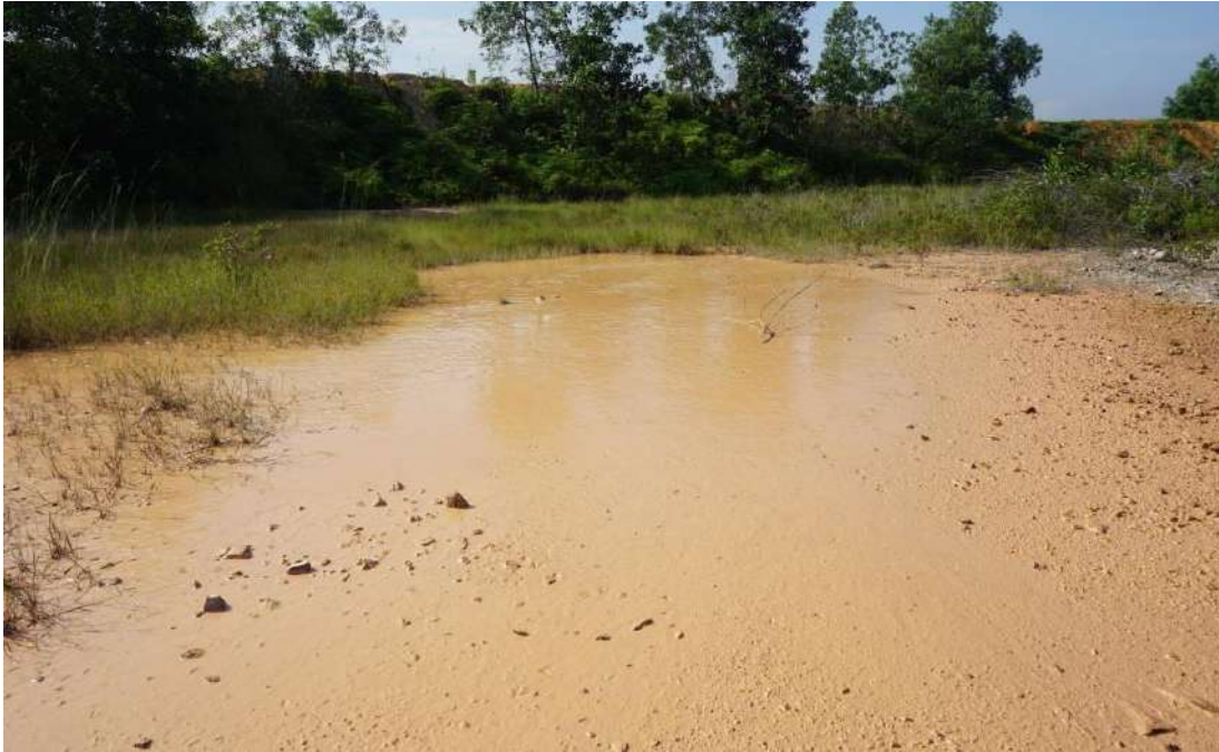
Figure 81: Several muddy areas are found uphill. A buffer zone or barrier is needed before further construction is done.
