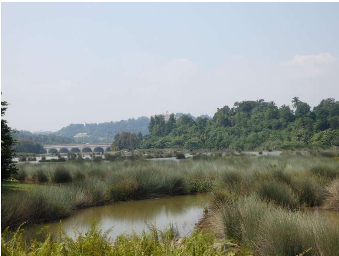
Figure 41: The surface flow constructed wetland with wetland plants to take up excessive nutrient at Putrajaya Wetlands. (Source: Wetlands International – Putrajaya Wetlands cells)
