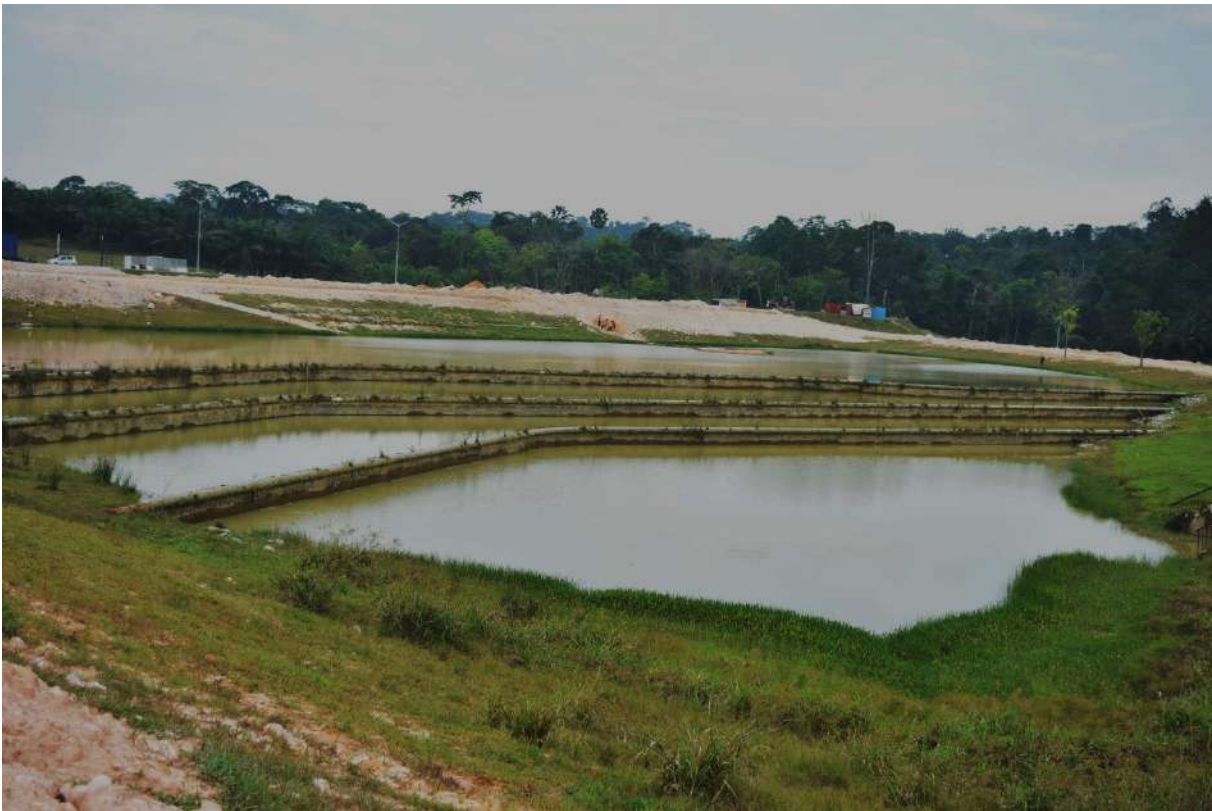
Figure 25: Elmina West Pond 10 – Upper Pond, showing terraced cascade.
