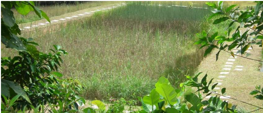
Figure 43: The horizontal sub-surface flow constructed wetlands where the water flows through the plants' roots and soil bed but does not rise above the soil surface. (Source: Wetlands International – the experimental plot at NAHRIM)
