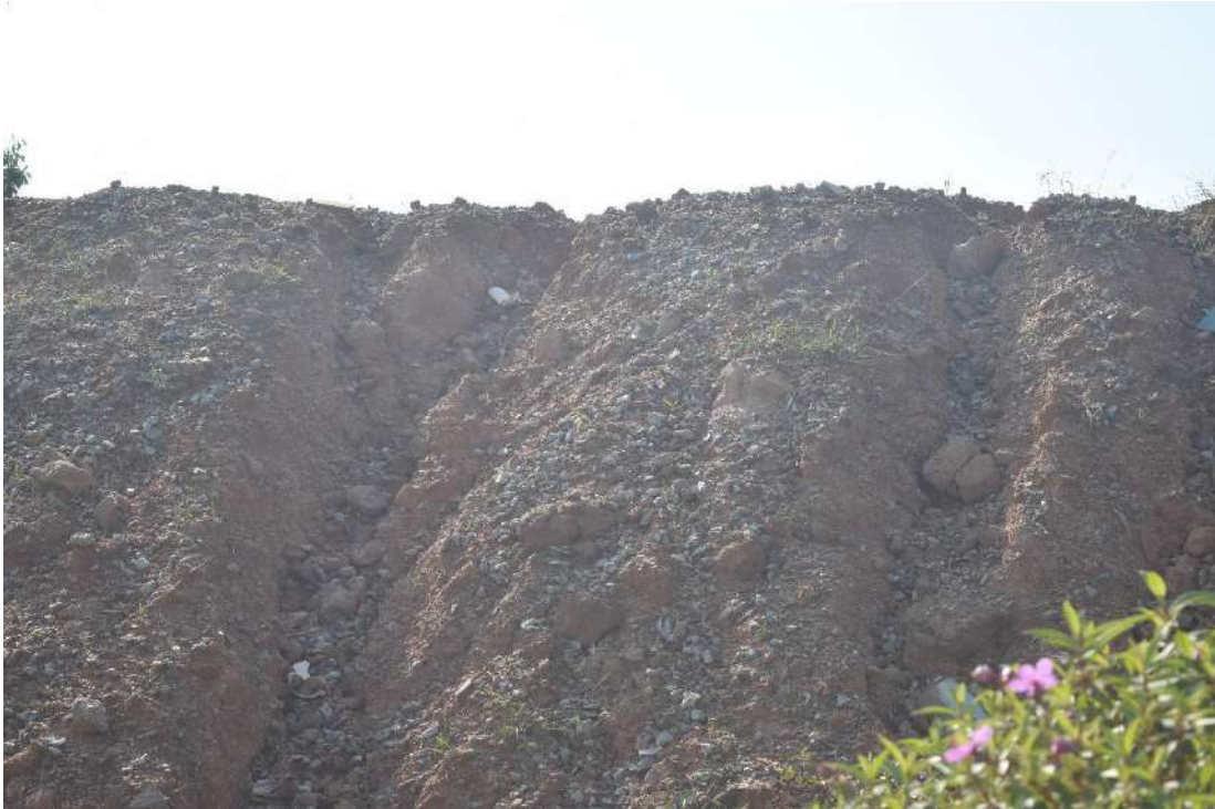
Figure 100: Sign of soil erosion sighted near Pond 4.
