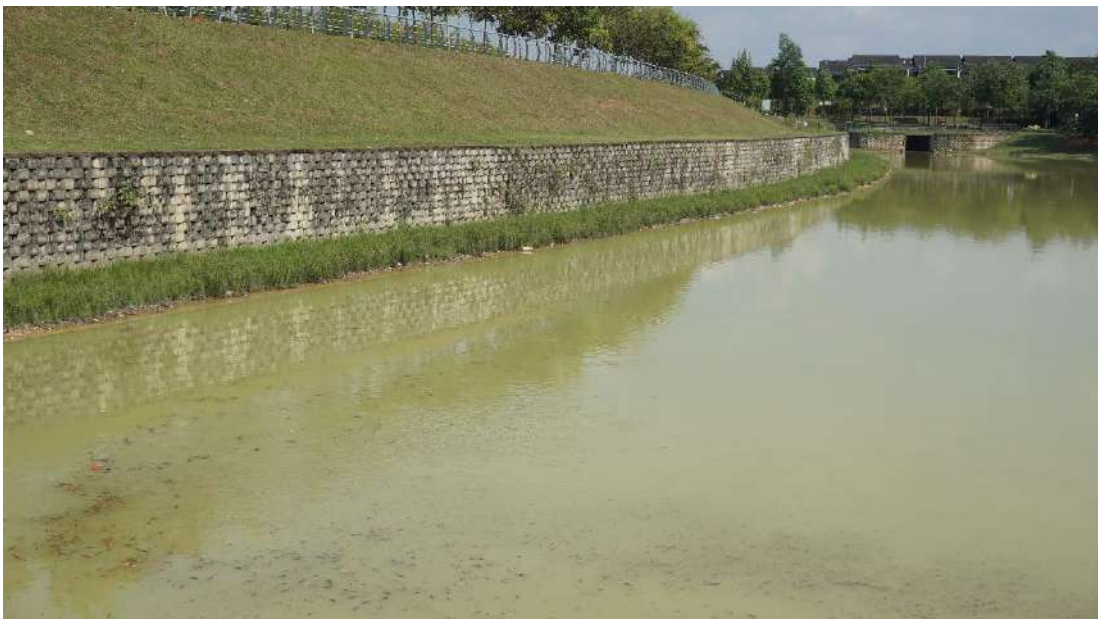
Figure 84: The steep slope of pond edge.
