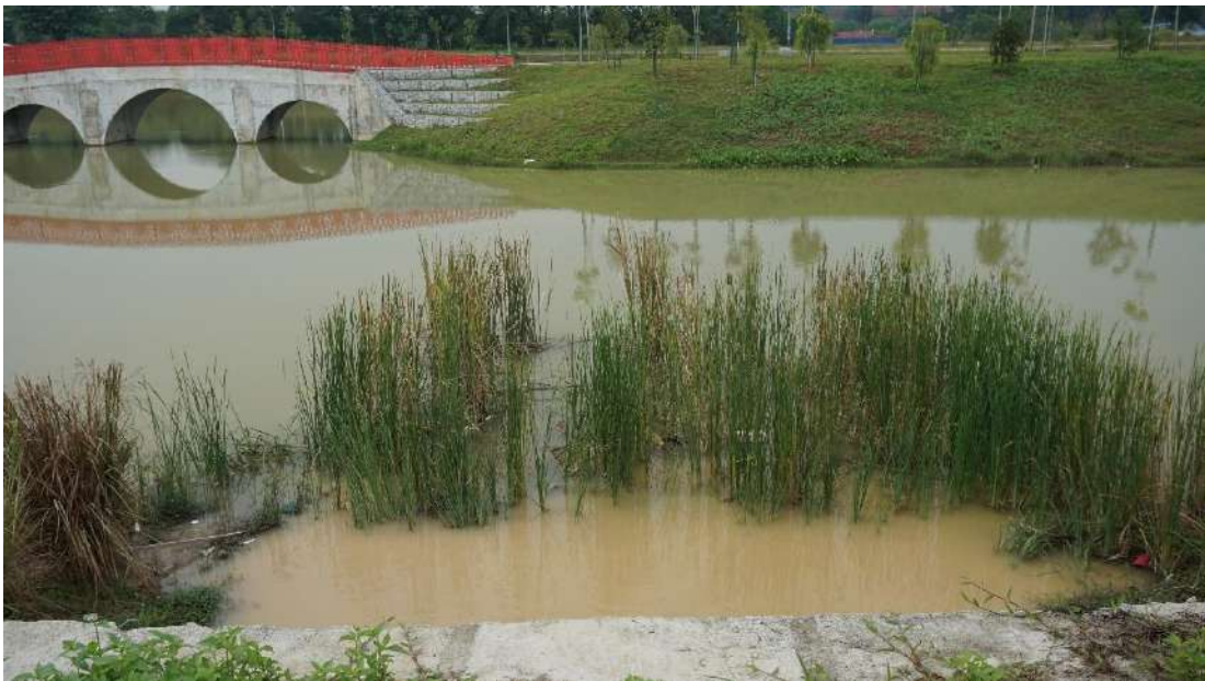
Figure 88: Existing plant filters sediments and rubbish from the runoff.
