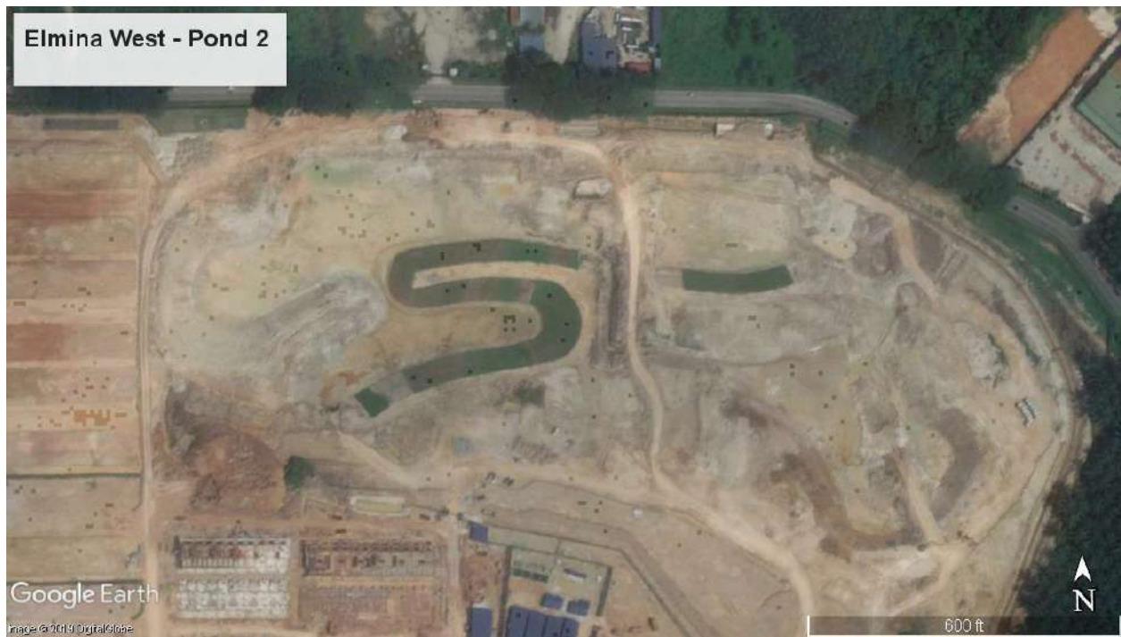
Figure 16: Google Earth satellite image (6-12-2017) of Elmina West Pond 2 under construction.
