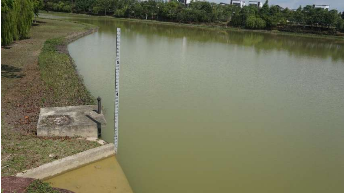
Figure 83: Low water level at Pond 5.
