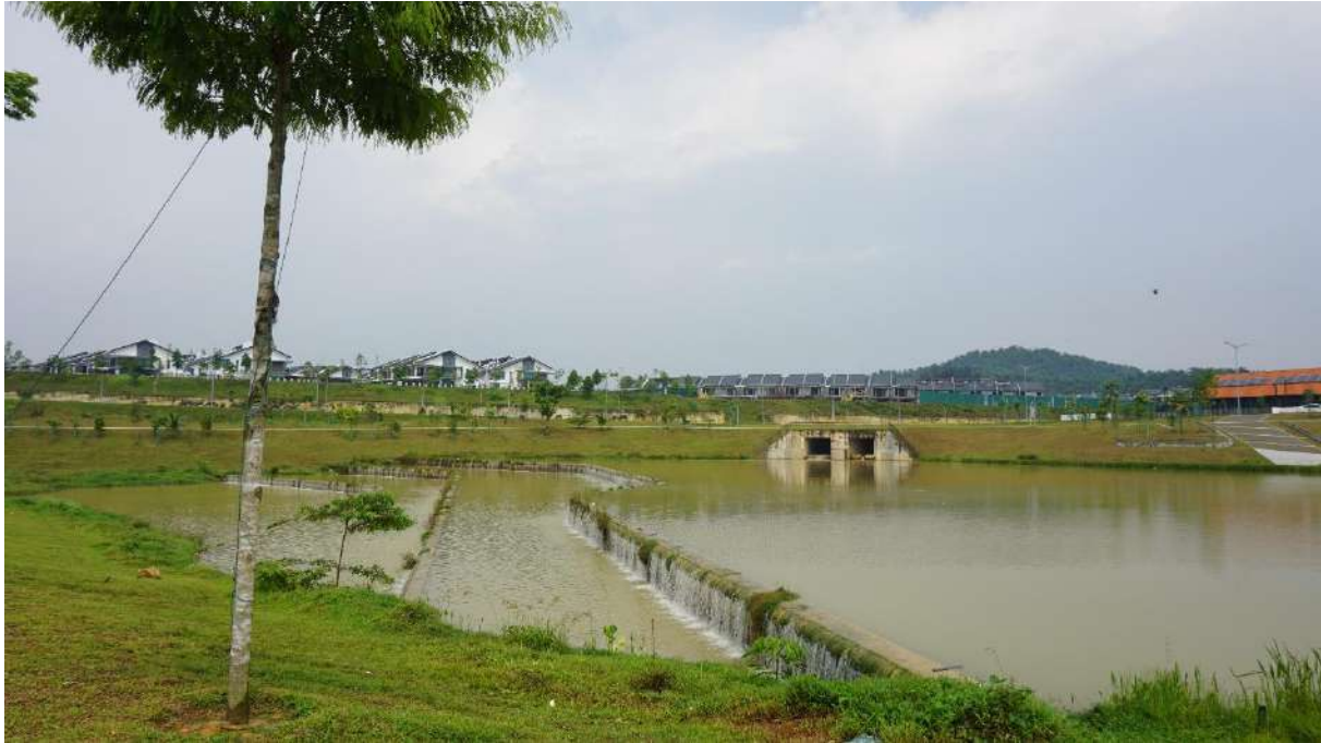
Figure 93: The current condition of Pond 10 during the survey.
