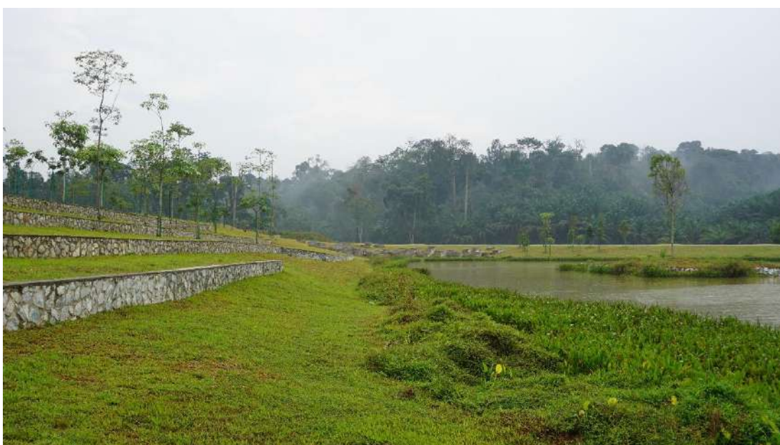
Figure 46: An example of consistent level for the top embankment level at Pond 10.
