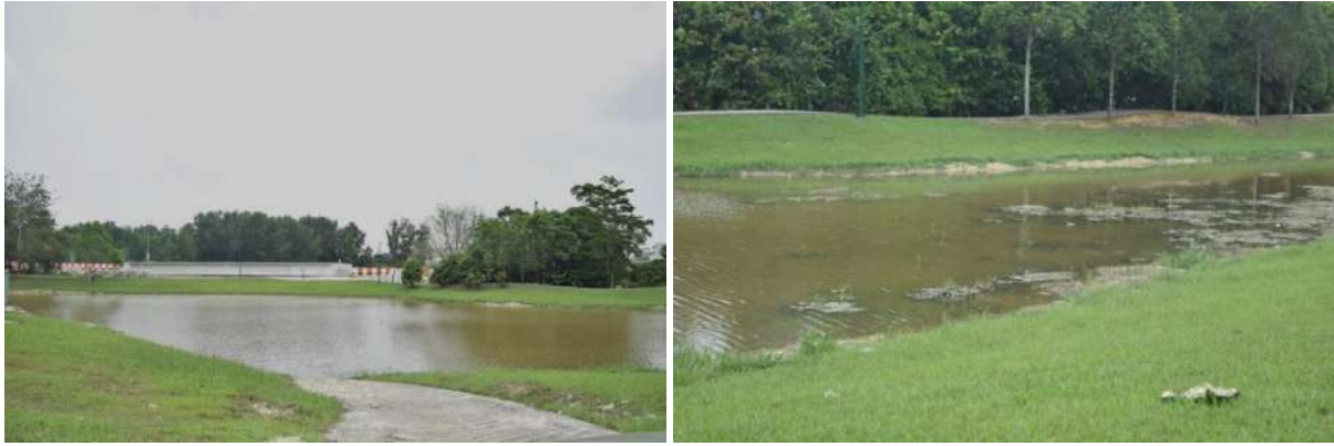
Figure 10: Current condition of Pond D, Denai Alam.
