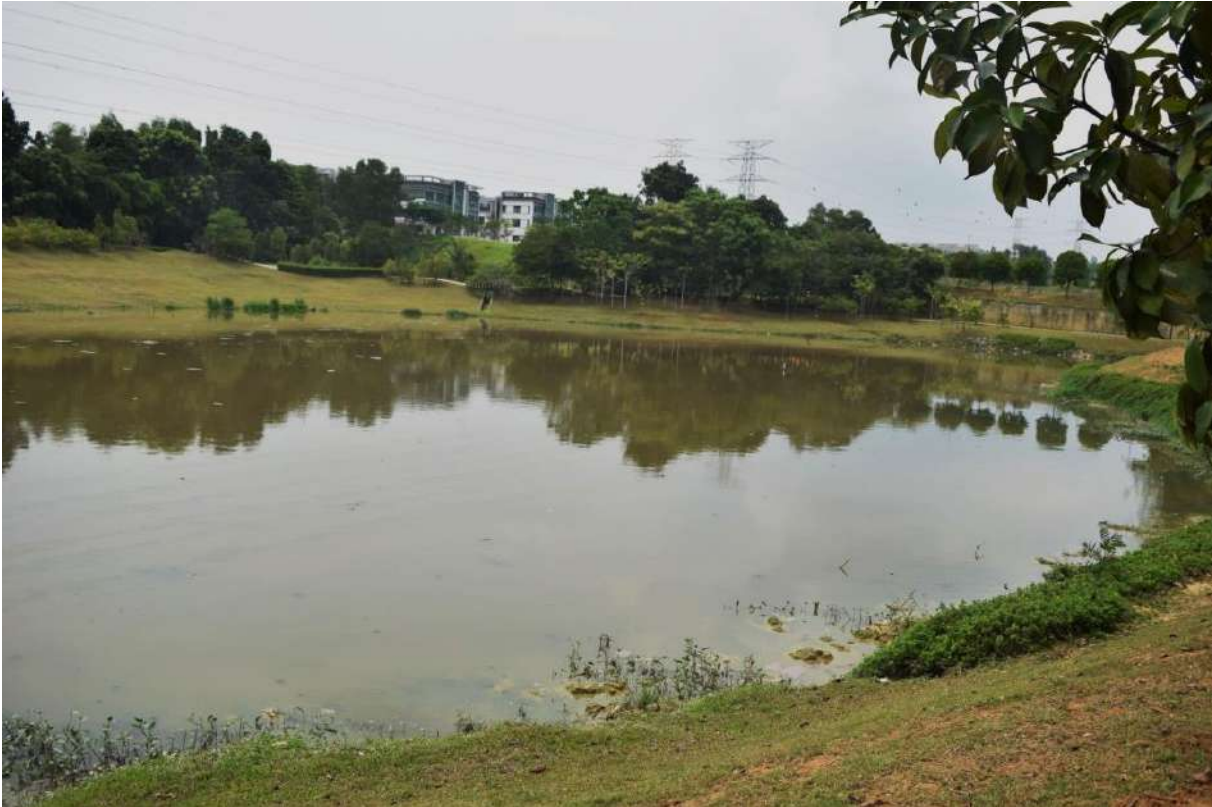
Figure 4: Current condition of Pond B.
