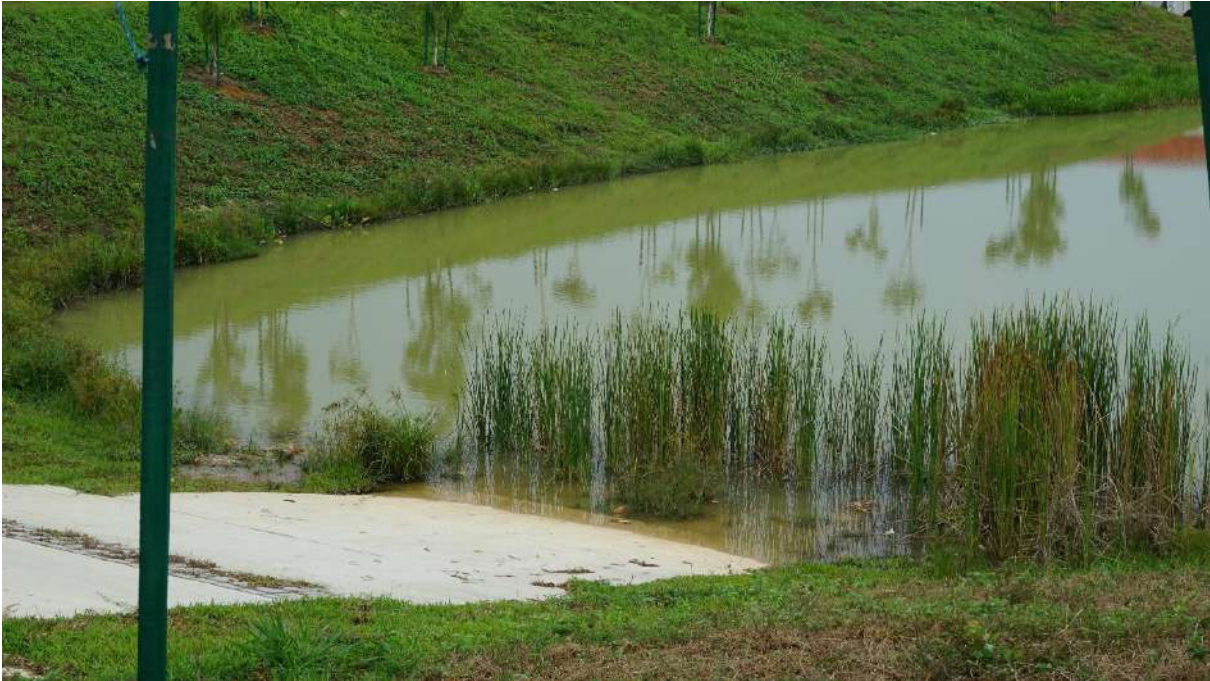
Figure 98: The concrete ramp for maintenance at Pond 2.
